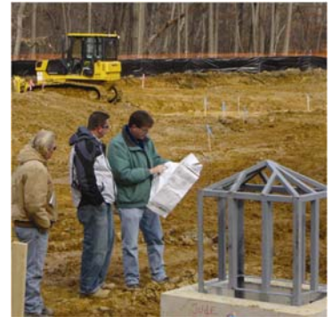
On-site CCR services
